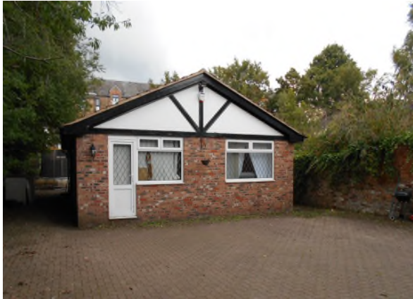
Existing bungalow: East-facing elevation
